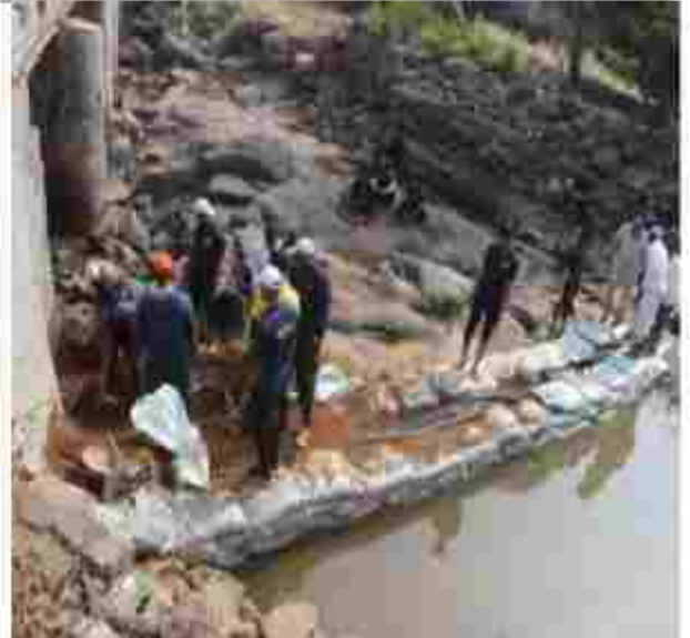
Construction of Vanrai Bandhara
